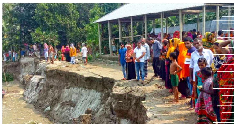
Flood waters erode banks further
